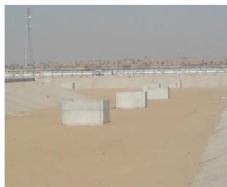
Photograph showing Recharge pit of storage capacity of (72,000 m 3 ) constructed in Mangala Processing Terminal (MPT), along with recharge shaft for artificial recharge of groundwater.
