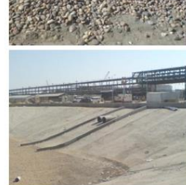
Photograph showing Recharge pit of storage capacity of (72,000 m 3 ) constructed in Mangala Processing Terminal (MPT), along with recharge shaft for artificial recharge of groundwater.
