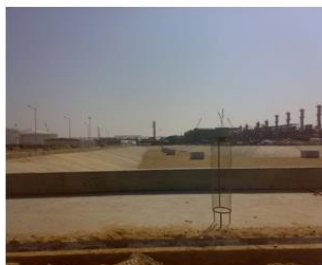
Photograph showing Recharge pit of storage capacity of (72,000 m 3 ) constructed in Mangala Processing Terminal (MPT), along with recharge shaft for artificial recharge of groundwater.
